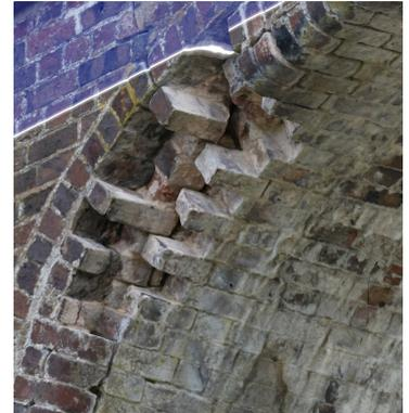
Figure 31: At least one broken brick face in here.
