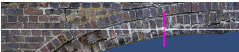
Figure 13: Plane shows that top of side hinge is on same level as crown intrados. A loose brick at the crown shows that there is no thrust at the intrados.
