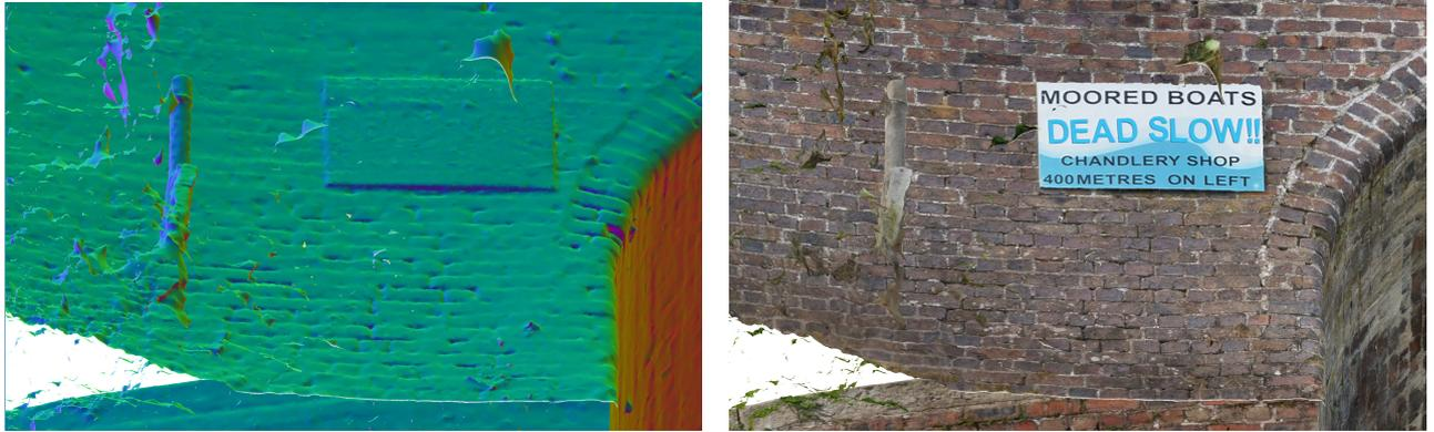
Figure 21: There are clear voids both in the wing wall and in the ring. In normal colour, and the empty joints are still visible but less striking.
