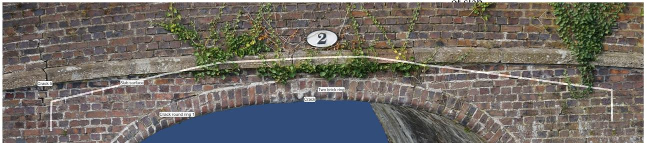
Figure 35: Eastern face showing extent of slab
