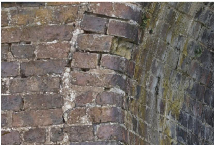
Figure 22: Do the gaps in the corner go round under the arch? This view shows that they don't. Note wide mortar indicating movement at back of ring, tight joints on the soffit, and snapped brick at the corner.
