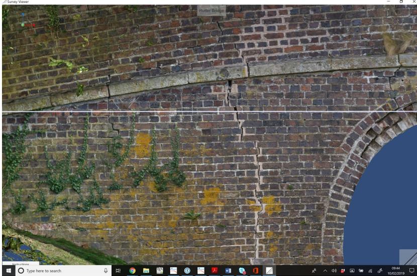
Figure 9: Closer view of left abutment face shows multiple vertical cracks with courses tilting backwards.
