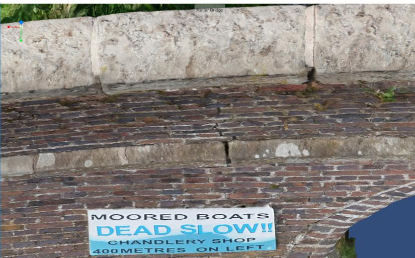
Figure 17: Inclined view of SLOW sign. I think that crack bifurcates and reaches both ends of the coping stone. This movement is caused by the twist in the bridge. The step is masked as a slew in a long stone at the parapet.
