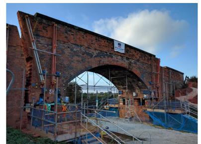
Figure 1: Moco Farm bridge, raised by 900mm
