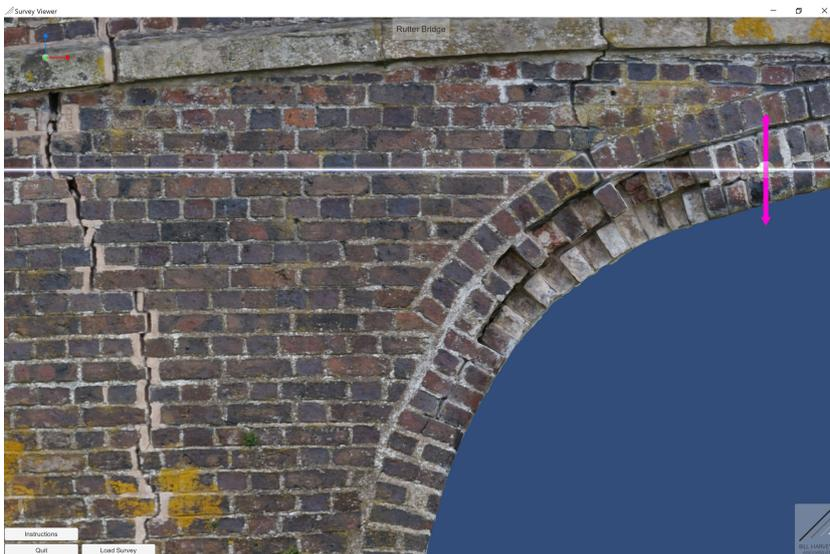
Figure 10: Close zoom of left abutment face shows that the course is curved.
