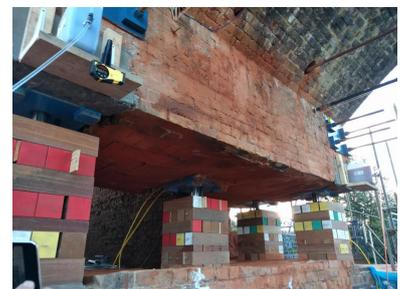
Figure 2: South abutment of Moco Farm bridge, raised by 900mm
