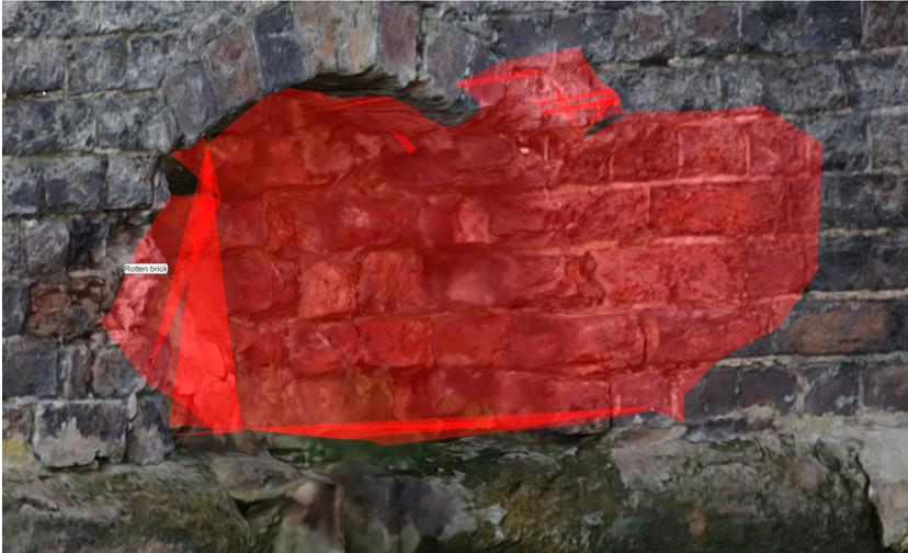
Figure 37: Stoplog hole detail showing 3D nature of tints. Careful examination of this view shows the steel channel to receive the stoplogs.
