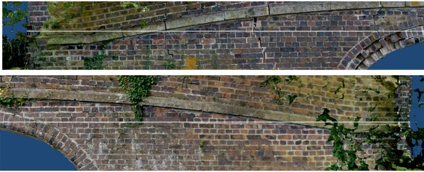
Figure 14: Same view, opposite sides of abutment, with the plane unmodified, shows a cross fall in the abutment.
