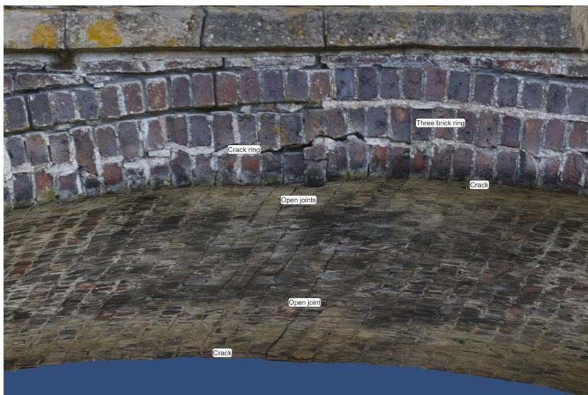
Figure 33: A closeup of the annotations near the crown.
